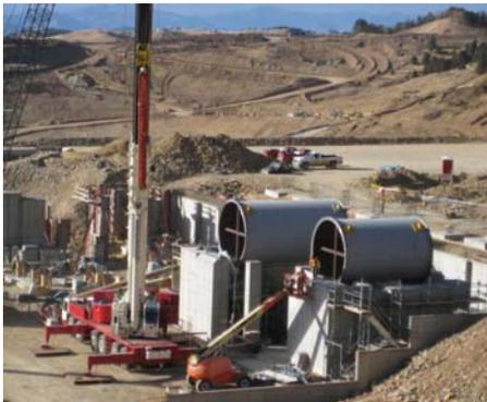
MLE2 project shells in place for rod mill (right) and ball mill (left).
