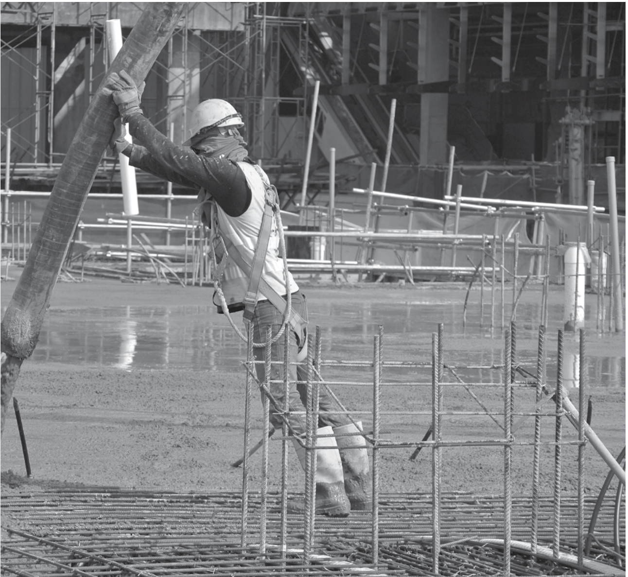
ZEAC head office under construction
