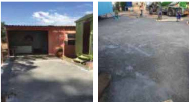
Concrete being delivered at Lerato Education Centre
