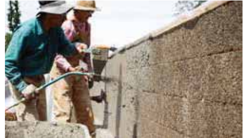
Plastering a wall
