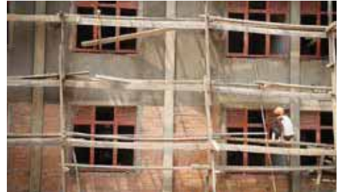
Rwanda construction Construction of student housing complex, Butare
