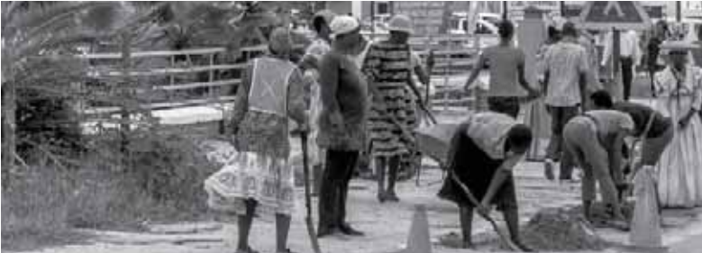
Maun, Botswana – women workers make road repairs
