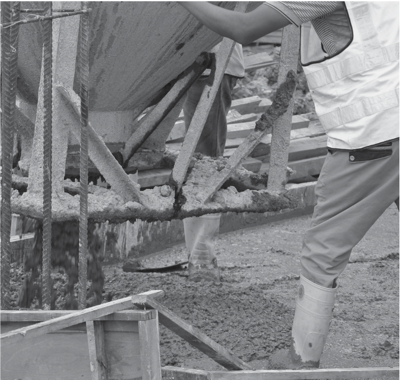
Likasi, school being built
