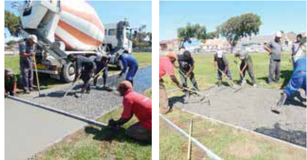
Constructing cricket pitches
