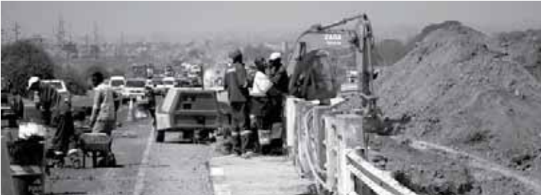
Bridge repair work, Harare
