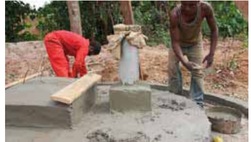
Building a new well in Bangadi, DRC
