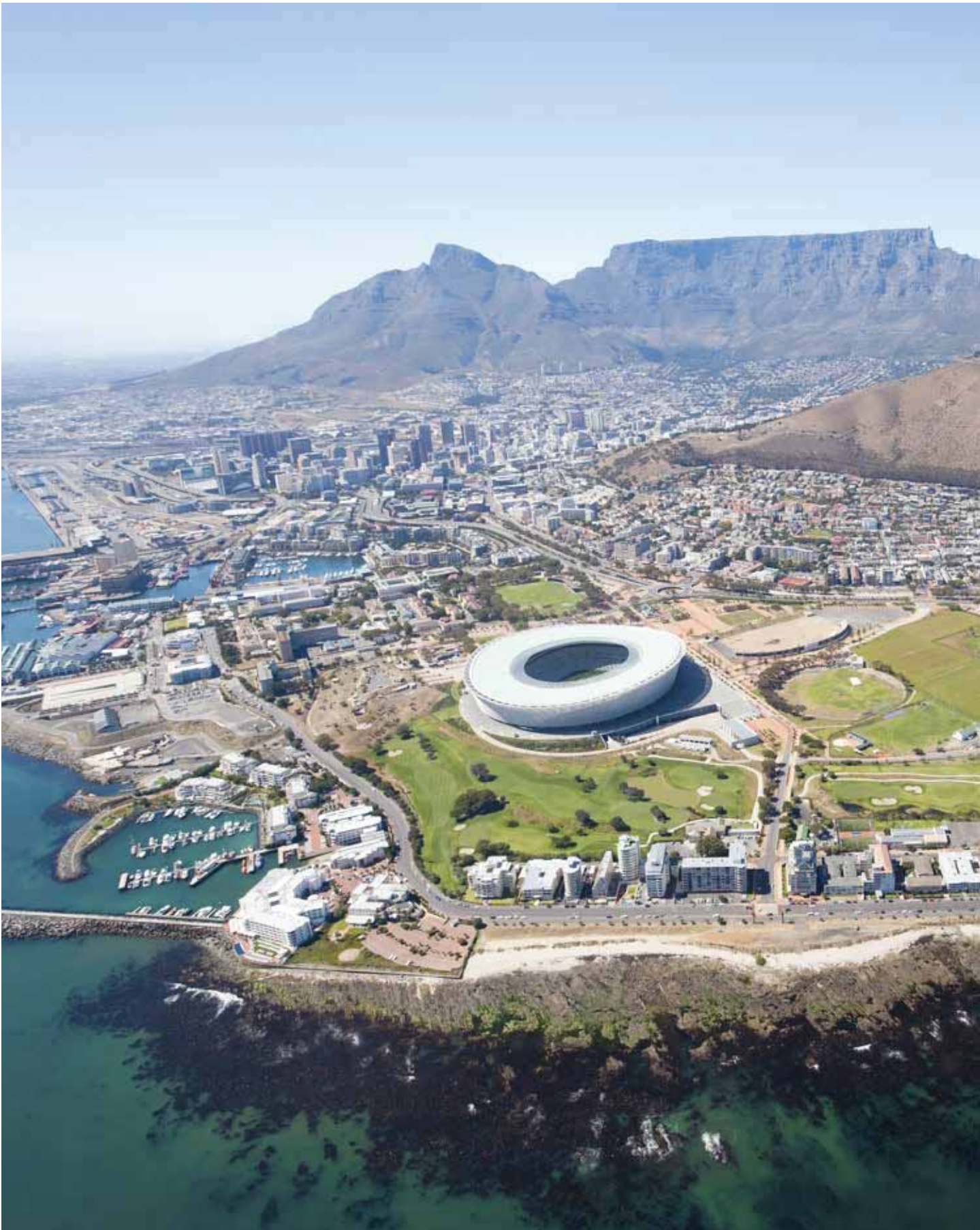
Aerial view of Green Point Stadium in Cape Town
