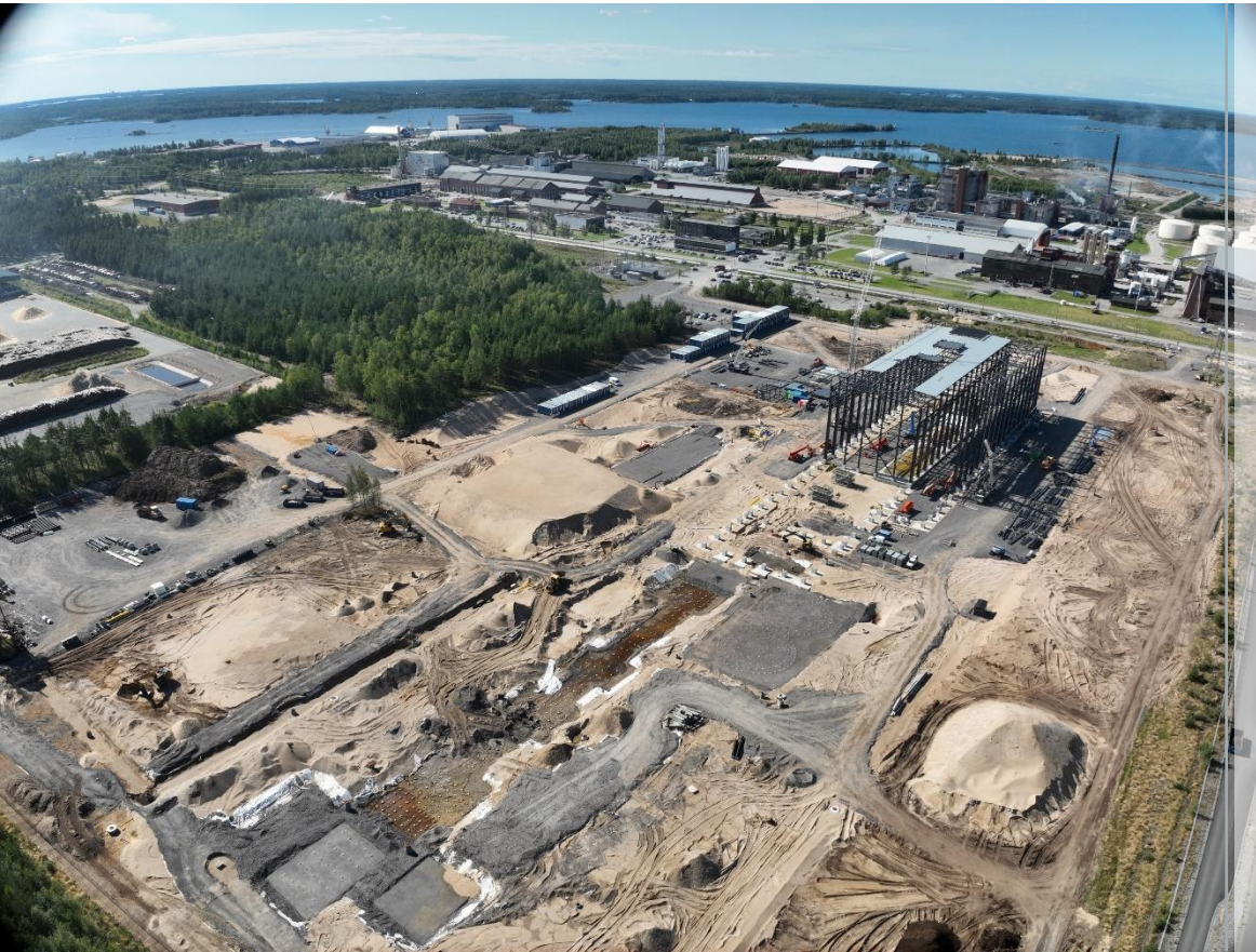
Aerial view of the construction at the Keliber lithium refinery August 2023 (credit: Tallqvist)
