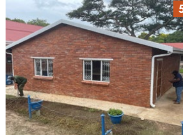
5 Upgrading of Sonop Primary School (Madibeng Local Municipality)
