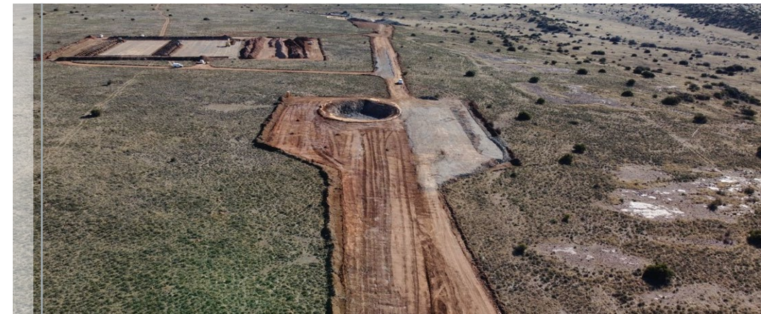
Aerial views of the construction at the Castle wind energy project during August 2023
