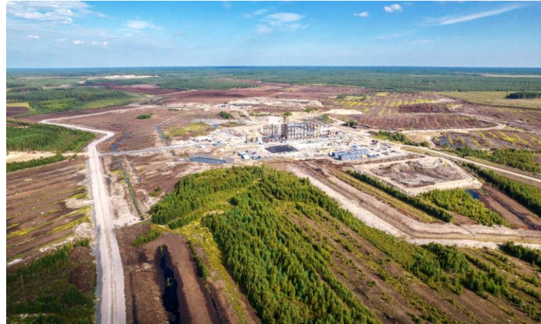
Päiväneva concentrator – earthworks commencing (9 Aug 2024)
