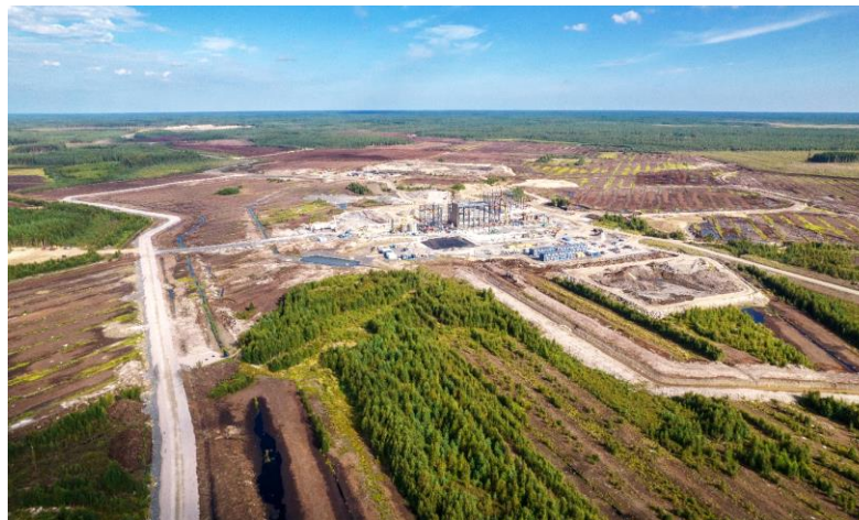
Päiväneva concentrator – earthworks commencing (9 Aug 2024)
