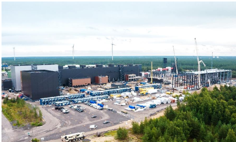
The lithium refinery in construction in Kokkola (10 Aug 2024)
