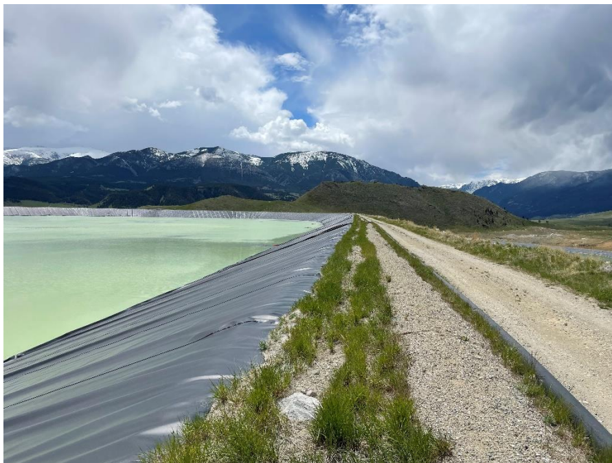
PHOTO 14 – Tailings delivery pipeline on embankment crest (2022).
