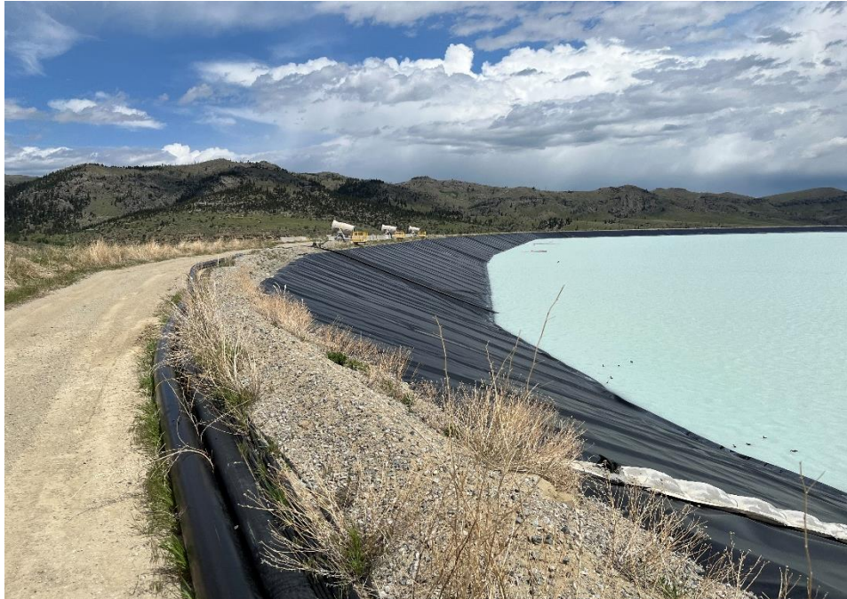
PHOTO 7 – West Embankment upstream slope with evaporators installed looking north (May 2024).
