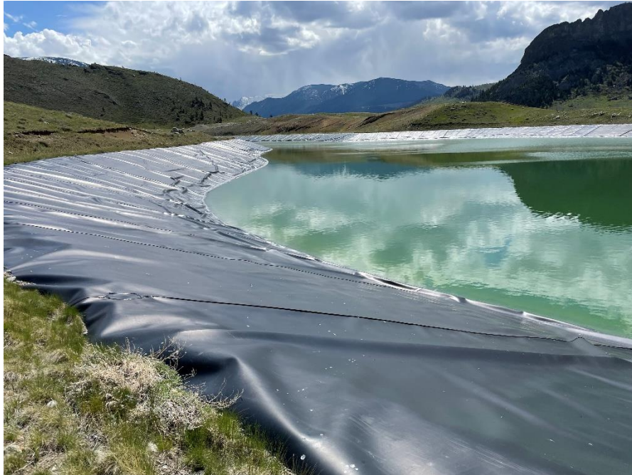
PHOTO 17 – North end of LAD Storage Pond (2022).
