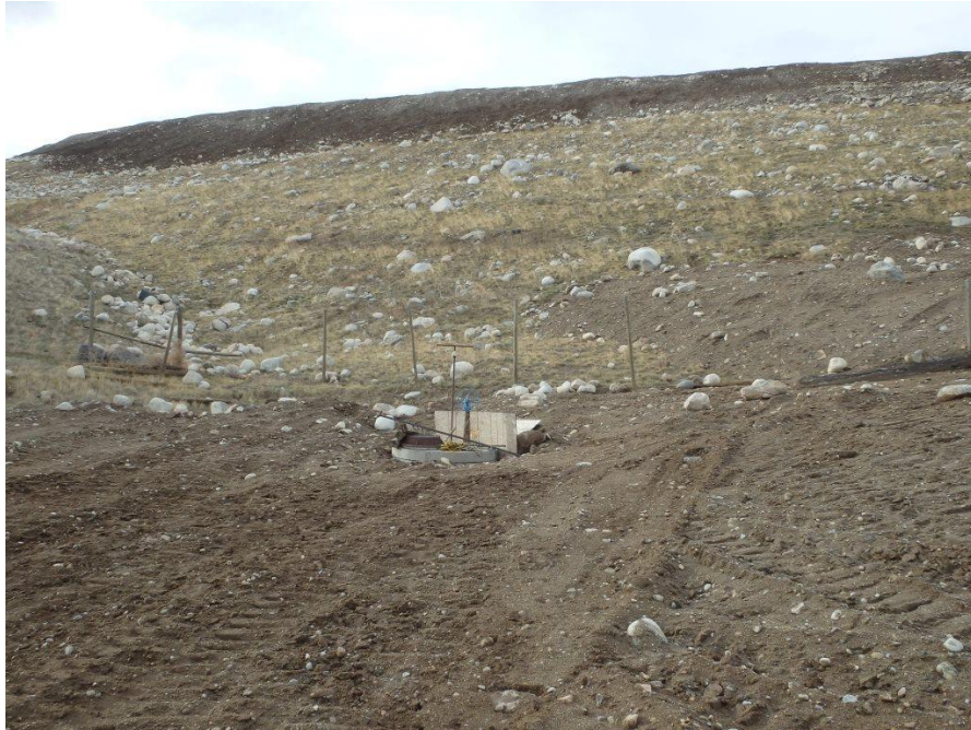
PHOTO 11 – Cell 2 Basin Underdrain Collection Sump (2015).
