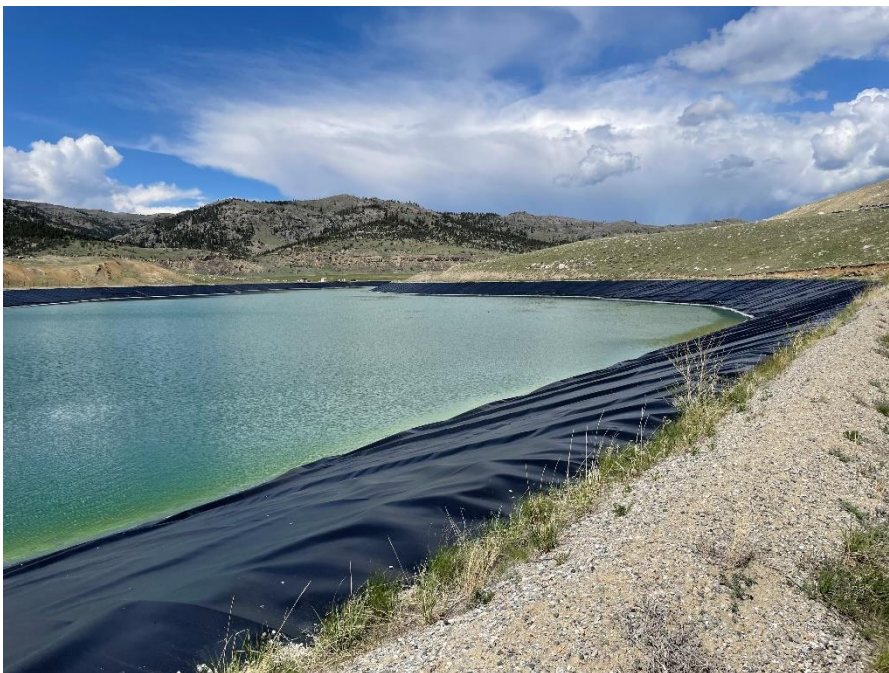
PHOTO 18 – South end of LAD Storage Pond (2022).
