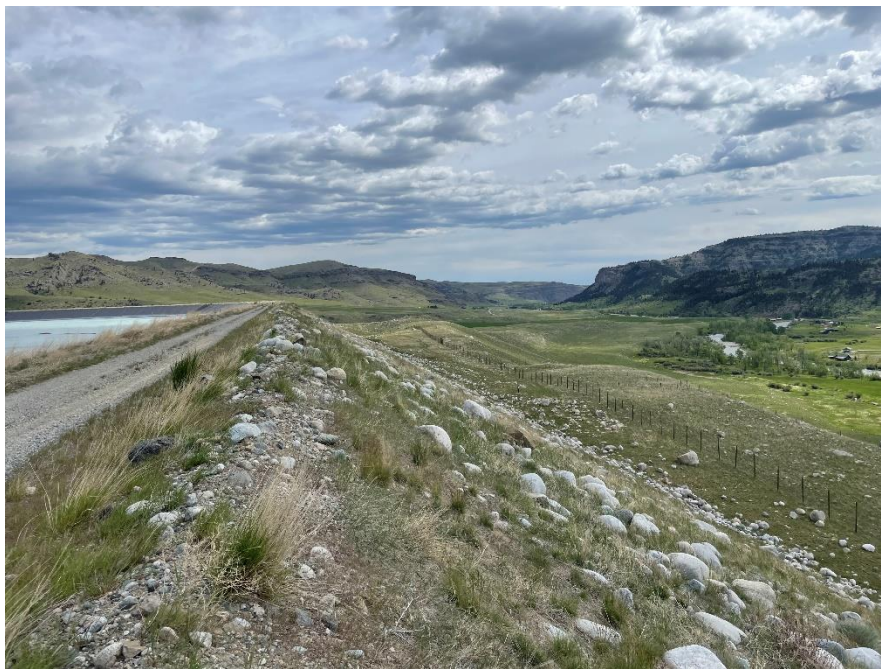
PHOTO 12 – East Embankment downstream slope looking north (May 2024).
