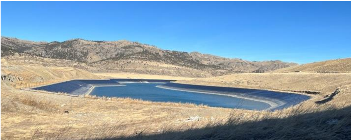
PHOTO 2 – Overview of LAD Storage Pond (January 2024).
