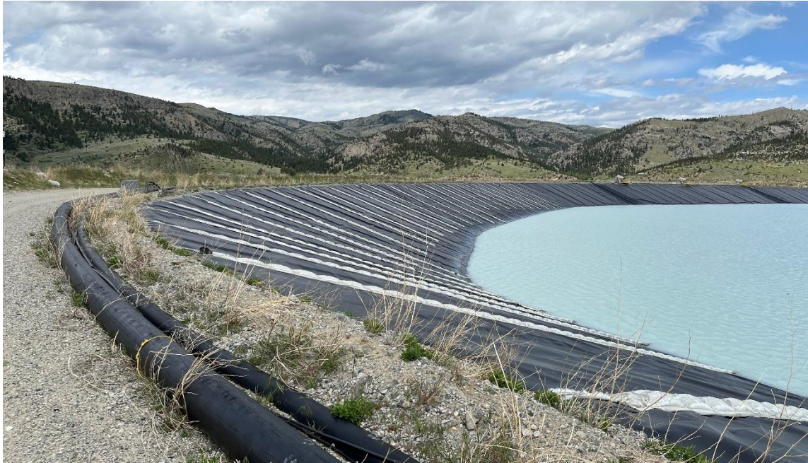
PHOTO 5 – Southwest Embankment upstream slope (May 2024).
