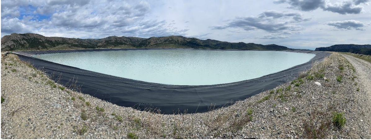
PHOTO 1 – Overview of Hertzler TSF (May 2024).
