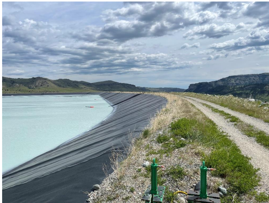
PHOTO 4 – East Embankment upstream slope looking north (May 2024).
