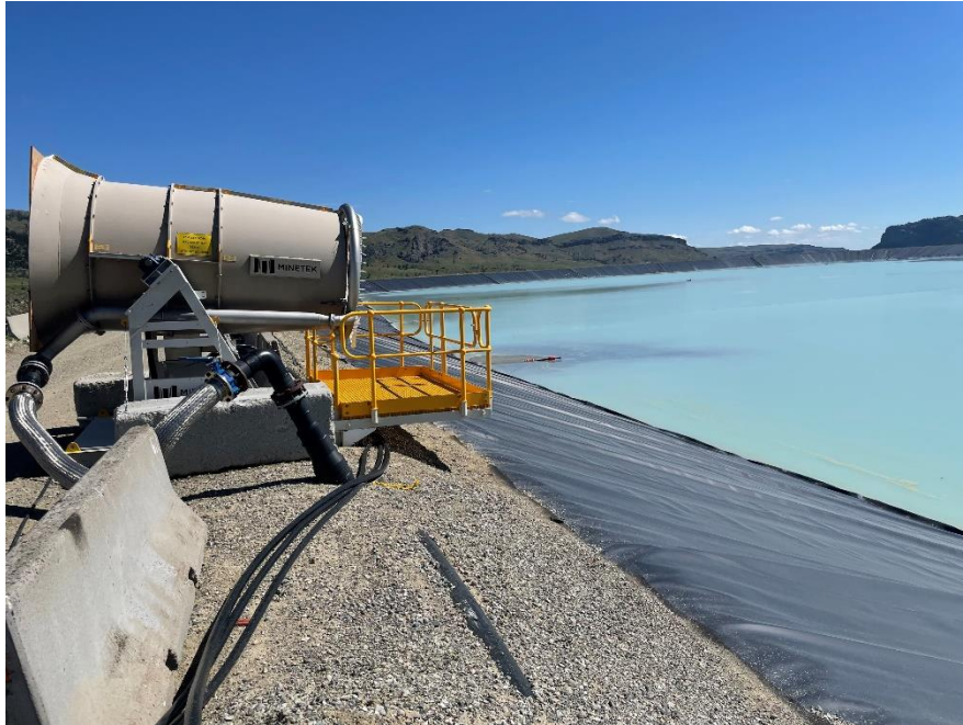
PHOTO 15 – Evaporator installation on West Embankment Crest (2022).
