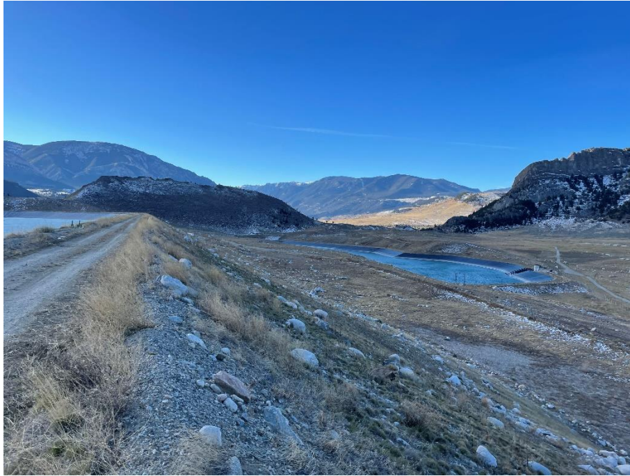
PHOTO 13 – West Embankment downstream (Nov. 2023).
