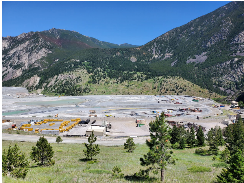
PHOTO 2 – Overview, Interim Cap, south end of TSF (June 2025).
