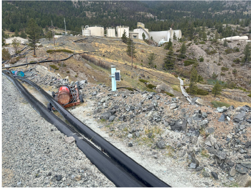
PHOTO 9 – Survey monument on North Embankment crest (April 2025).
