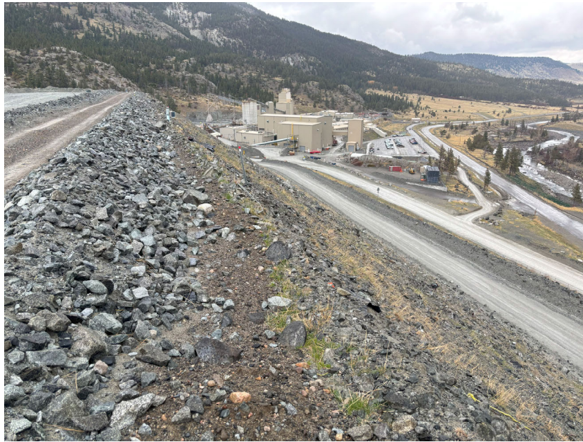
PHOTO 5 – Northeast Embankment downstream slope (April 2025).
