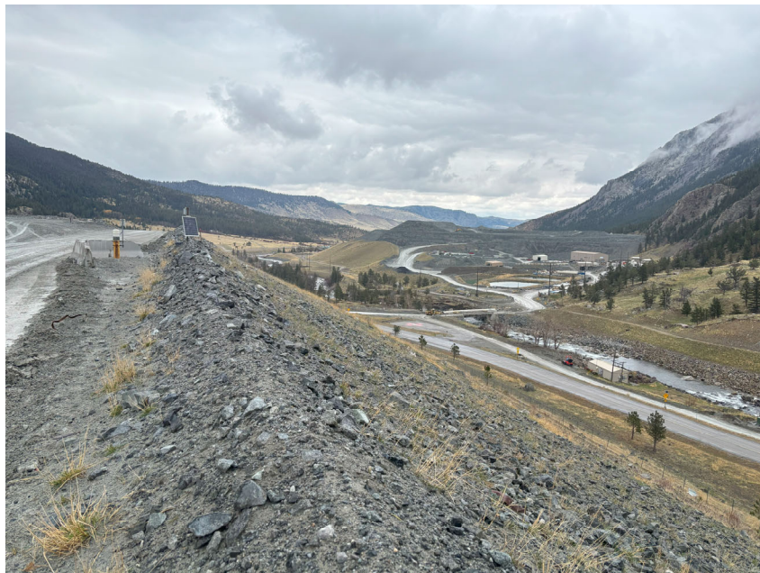
PHOTO 6 – East Embankment downstream slope (April 2025).
