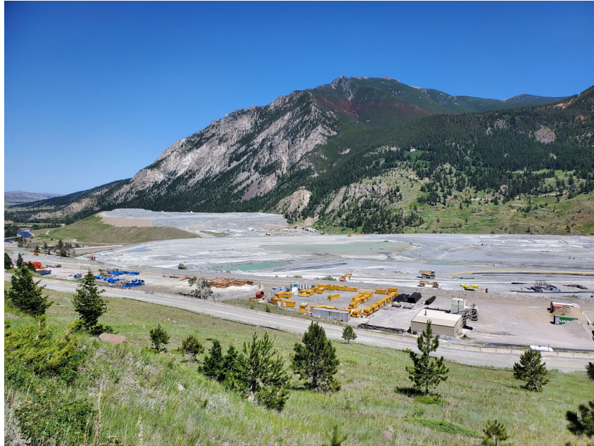
PHOTO 1 – Overview, Interim Cap construction progress, north end of TSF (June 2025).
