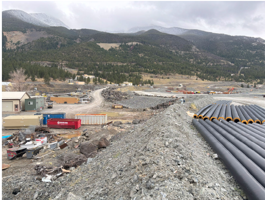
PHOTO 7 – South Embankment and Overflow Swale (April 2025).
