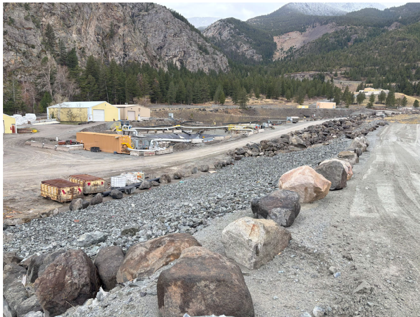
PHOTO 8 – Overflow Swale outlet, riprap remains to be installed (April 2025).
