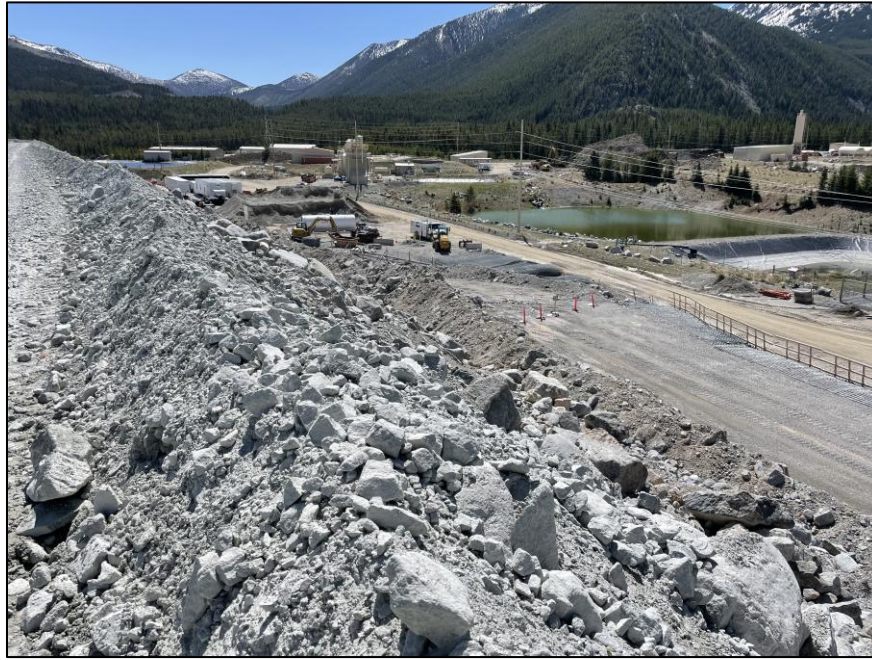
PHOTO 7 - South Embankment downstream slope, looking southwest (May 2024).
