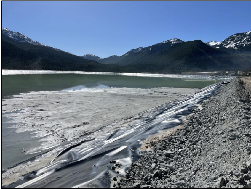
PHOTO 5 - Southwest Embankment looking southeast (May 2024).
