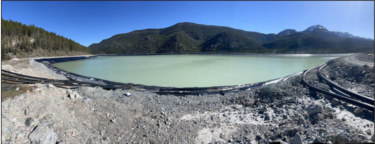
PHOTO 1 - TSF overview from South Embankment corner looking north (May 2024).
