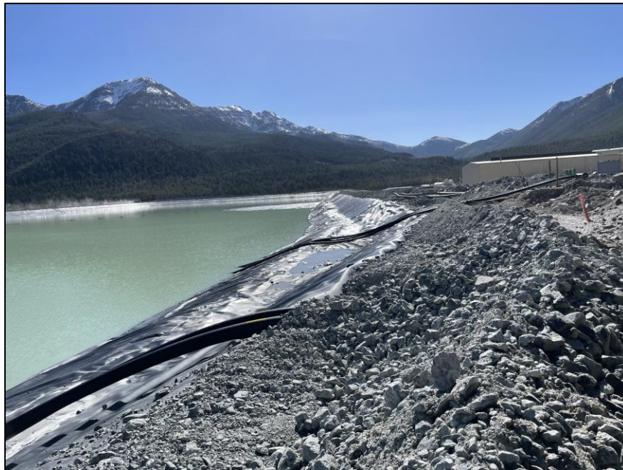
PHOTO 8 - South Embankment upstream slope looking east (May 2024).
