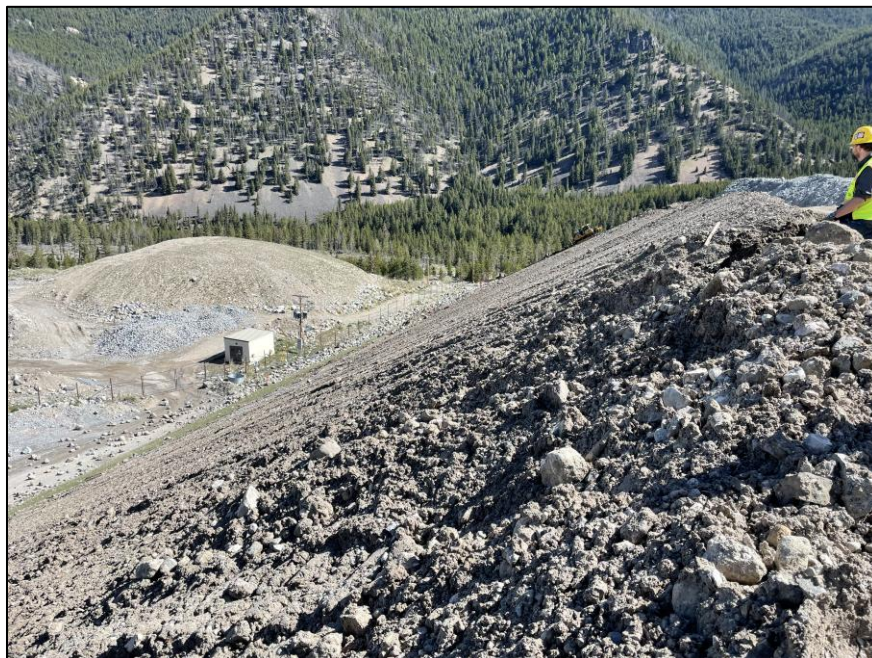
PHOTO 10 – West Embankment downstream slope, looking north (May 2024).
