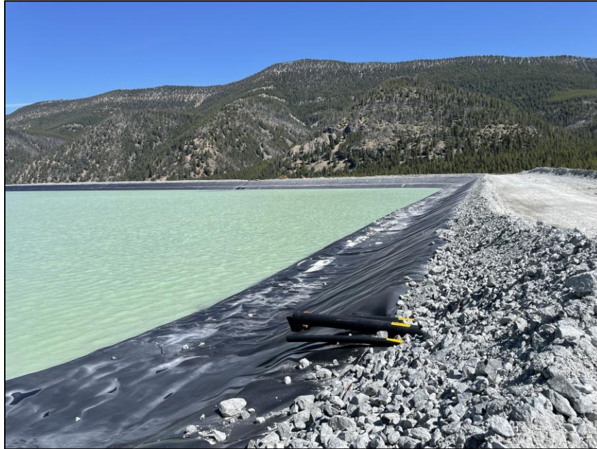
PHOTO 9 - East Embankment upstream slope looking north (May 2024).
