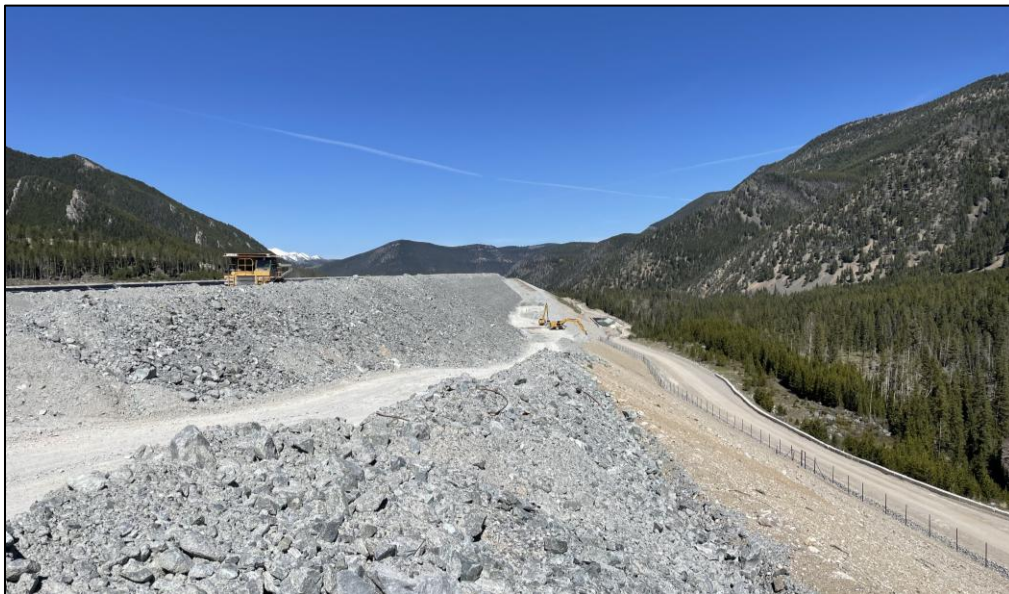
PHOTO 2 - North Embankment downstream slope looking northwest (May 2024).
