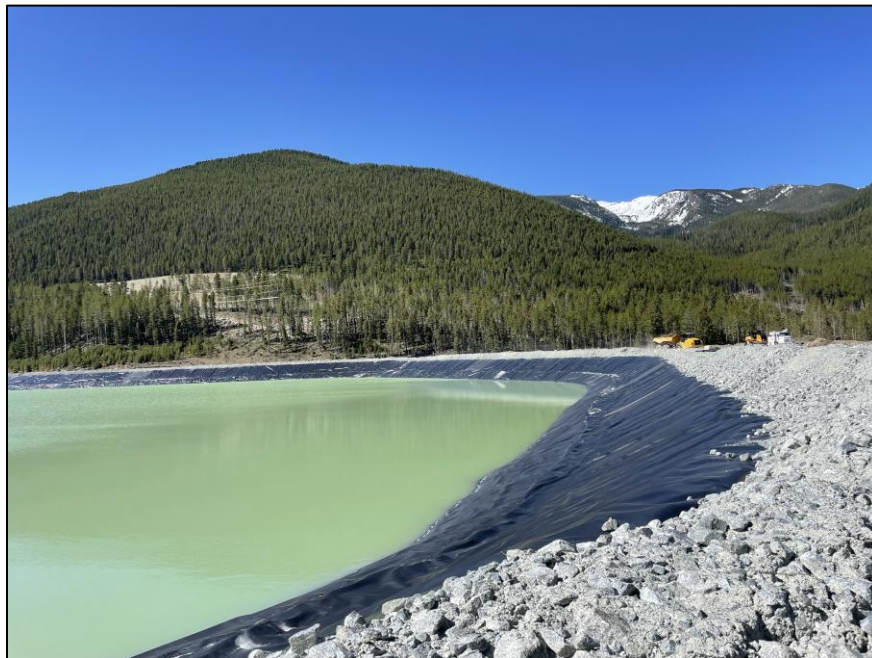
PHOTO 4 - West Embankment upstream slope, looking south (May 2024).
