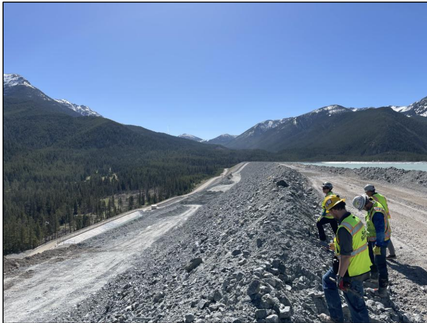
PHOTO 12 - North Embankment, Stage 6 ROM rockfill placement, looking east (May 2024).
