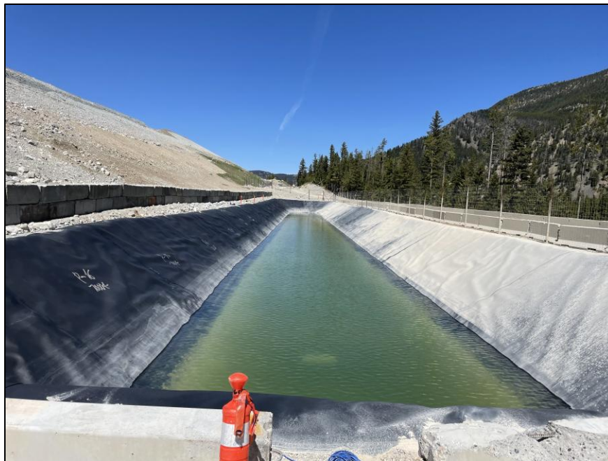
PHOTO 14 – Relocated Embankment Underdrain Collection Pond looking west (May 2024).
