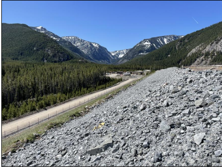
PHOTO 11 - East Embankment, Stage 6 ROM rockfill and surface soil placement on outer slope, looking south (May 2024).
