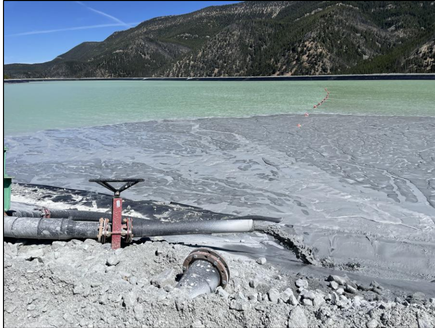
PHOTO 13 – Tailings Discharge line from the Southeast Embankment, looking east (May 2024).
