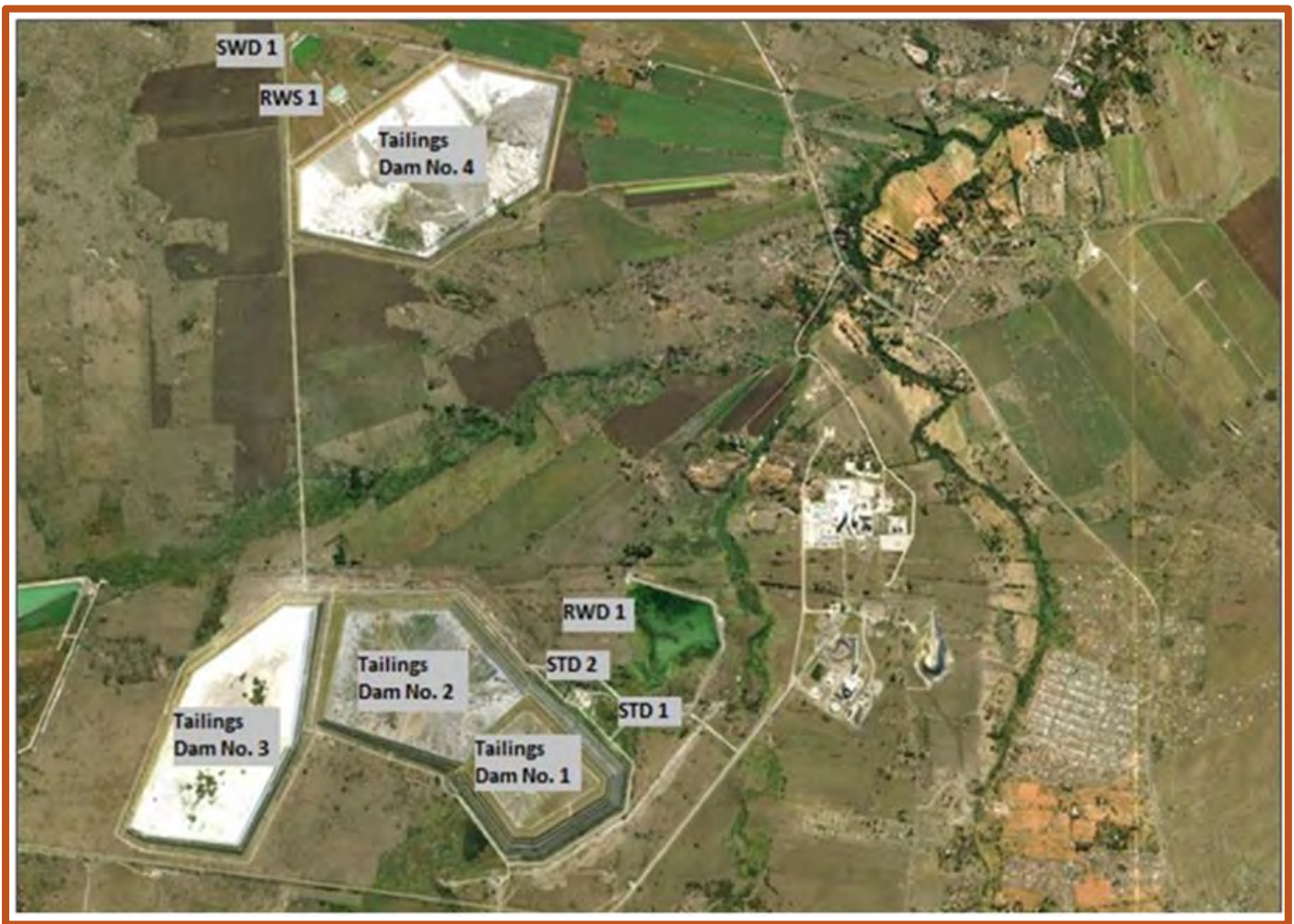
Figure 1: Layout of Karee Tailings Dam Complex
