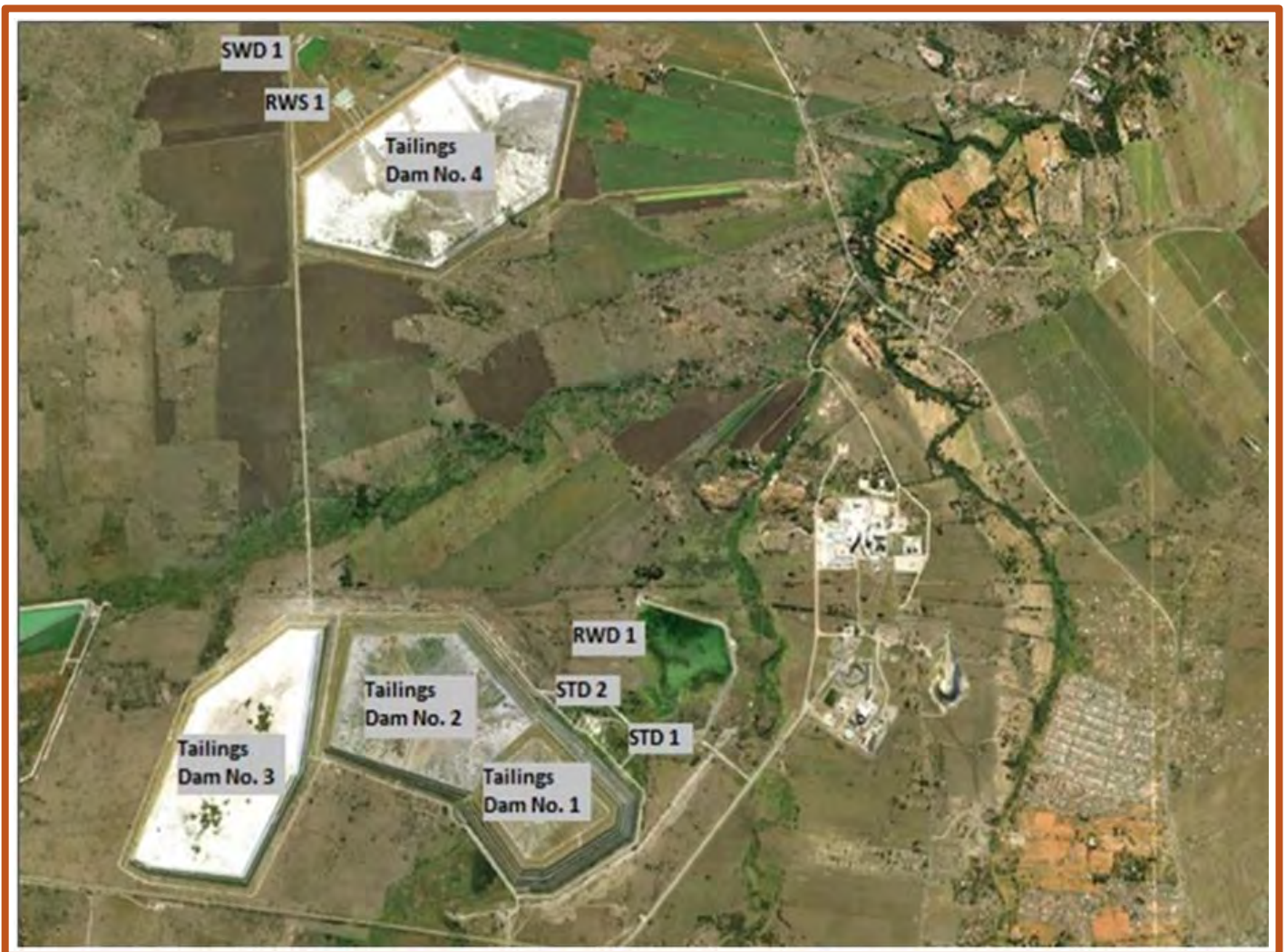
Figure 1: Layout of Karee Tailings Dam Complex
