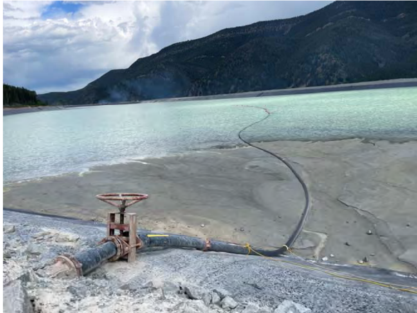
PHOTO 13 – Floating Tailings Discharge line from the Southwest embankment, looking north.
