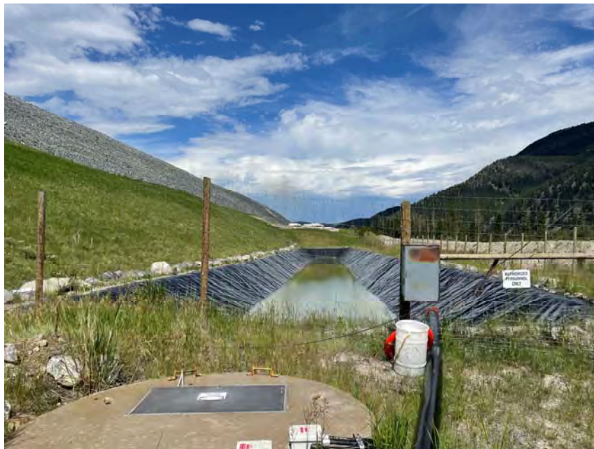
PHOTO 14 - Embankment Underdrain Collection Pond looking west.
