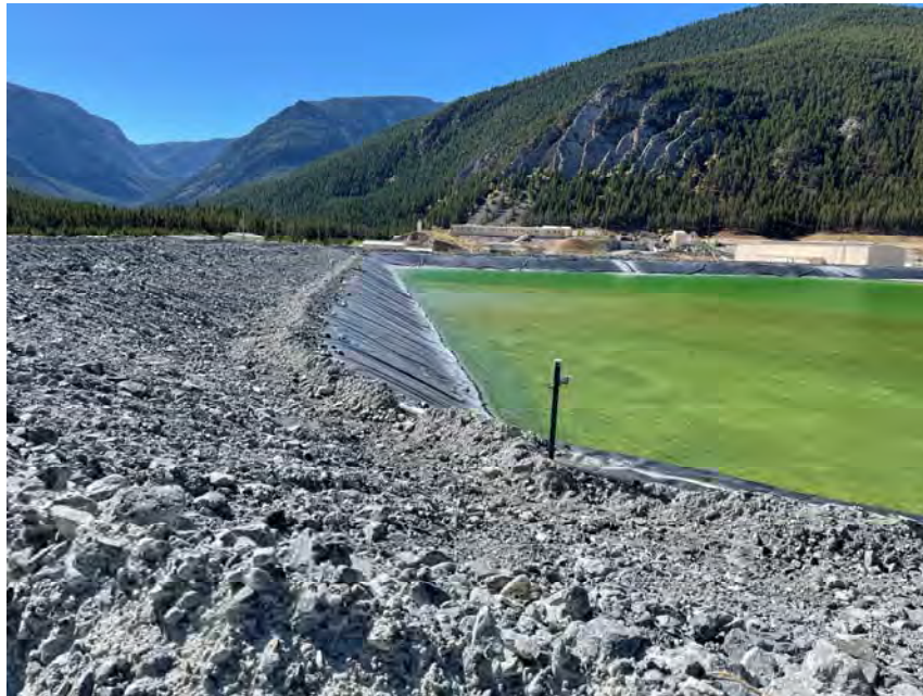
PHOTO 9 - GPS survey monument on East Embankment crest.
