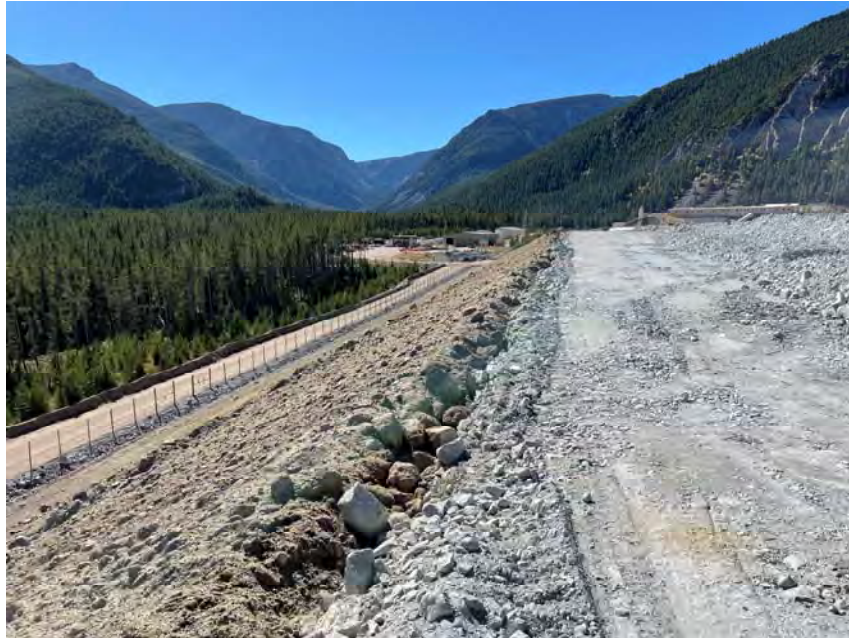
PHOTO 11 - East Embankment, Stage 6 ROM rockfill and surface soil placement on outer slope, looking south.
