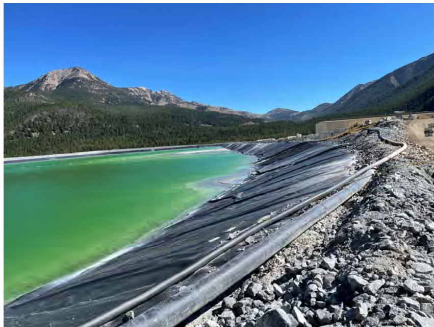
PHOTO 6 - Upstream slope of Southwest Embankment with reclaim water pipelines.
