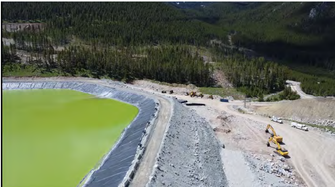
PHOTO 4 - West Embankment crest and upstream slope, looking south. Evaporators located on upstream embankment crest.
