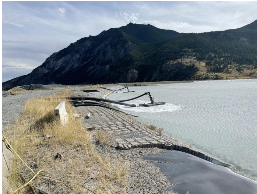
PHOTO 5 – Water reclaim and discharge pipework at the north end of the impoundment (Sept. 2022).
