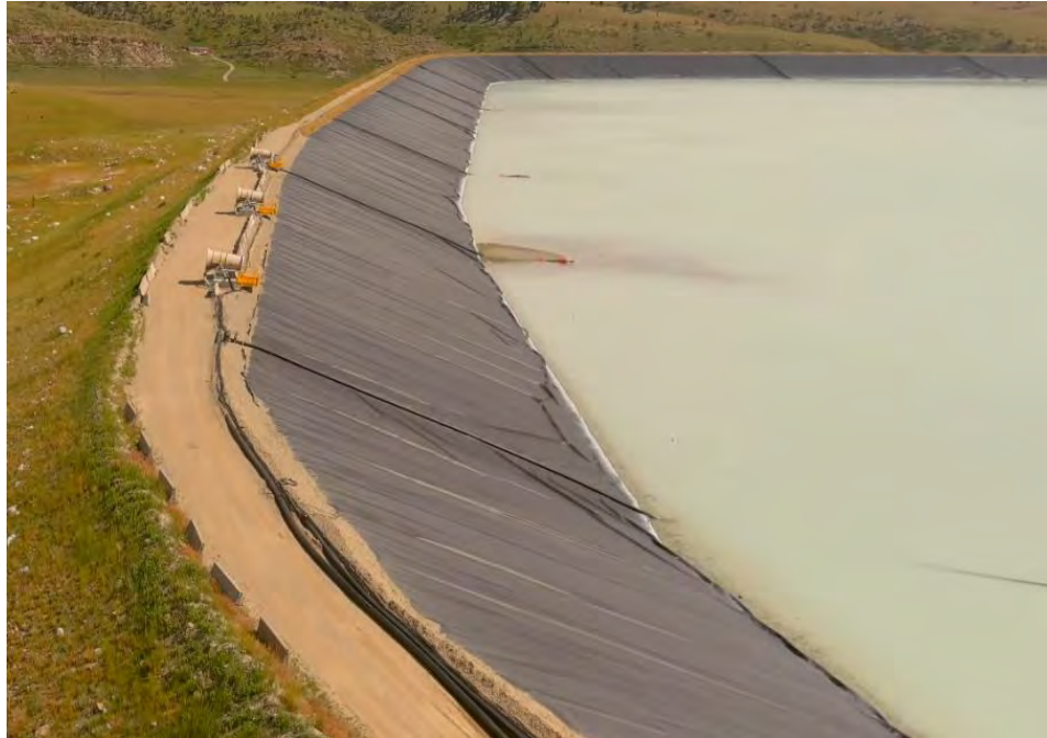
PHOTO 7 – West Embankment upstream slope with evaporators installed (2022).
