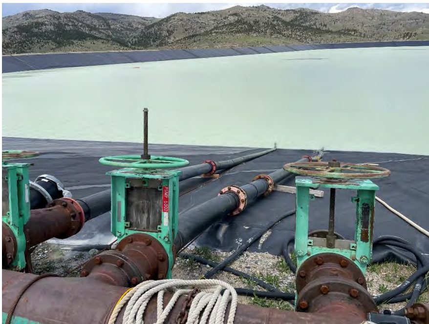
PHOTO 16 – Water reclaim manifold and pipework (2022).
