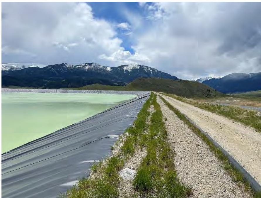
PHOTO 14 – Tailings delivery pipeline on embankment crest (2022).
