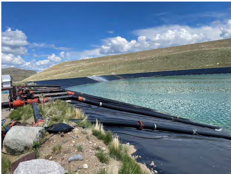
PHOTO 20 – LAD Storage Pond reclaim pipework and pumps (2022).
