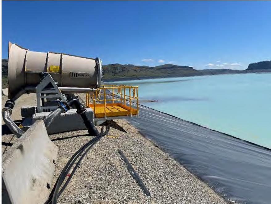
PHOTO 15 – Evaporator installation on West Embankment Crest (2022).
