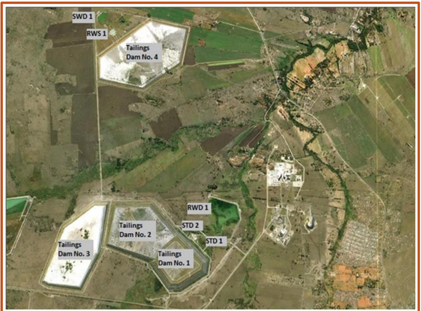
Figure 1: Layout of Karee Tailings Dam Complex
