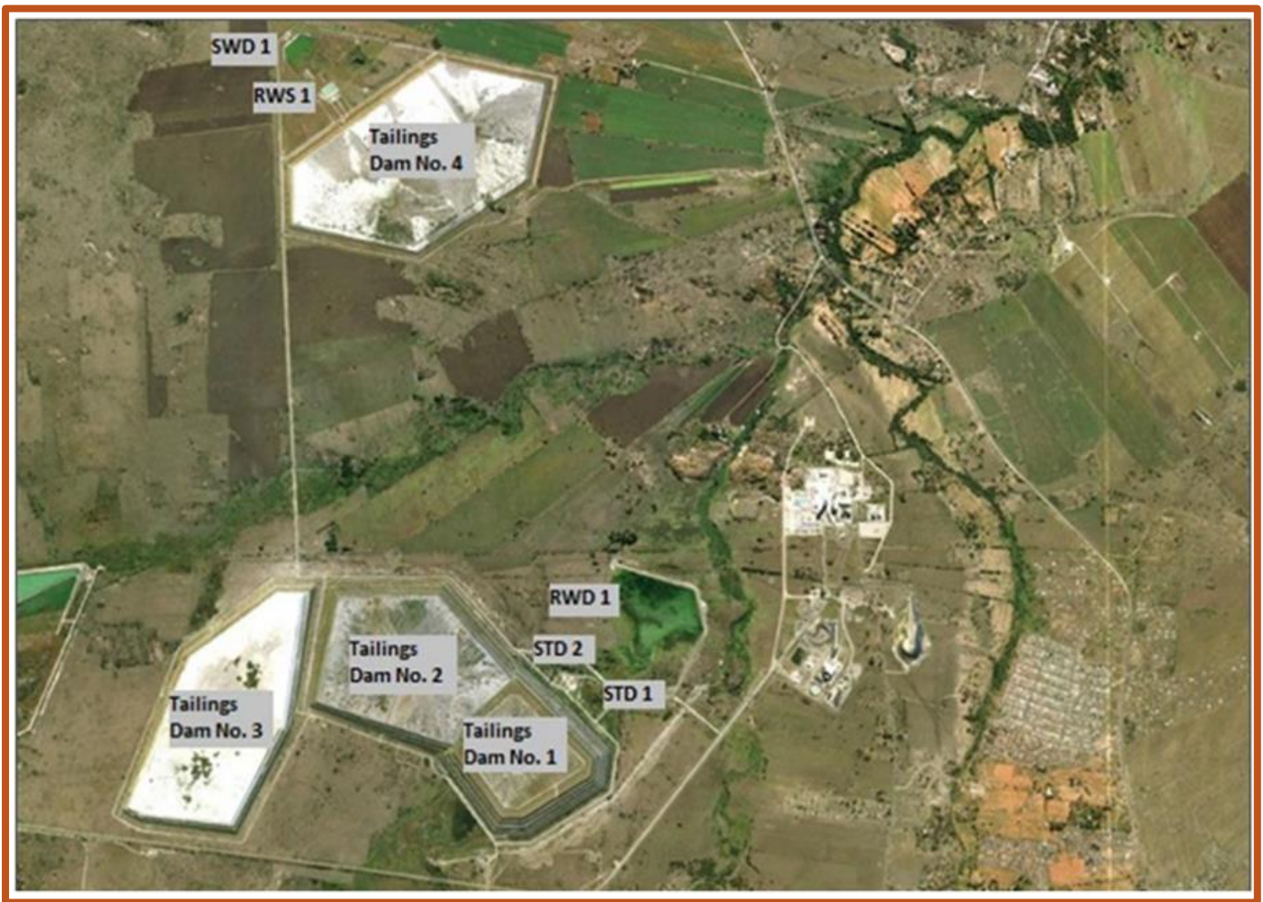
Figure 1: Layout of Karee Tailings Dam Complex
