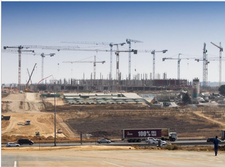
Mall of Africa under construction, Waterfall City (2014)
