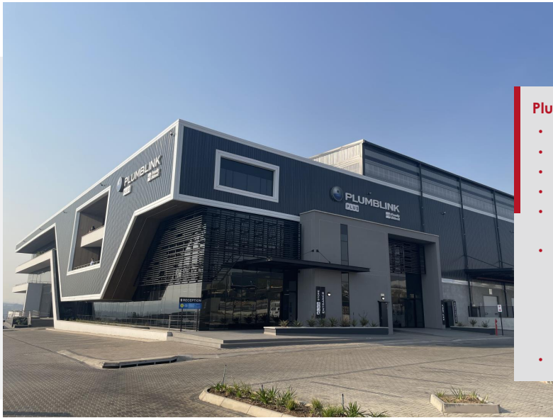
Plumblink head office and distribution centre, Waterfall City
