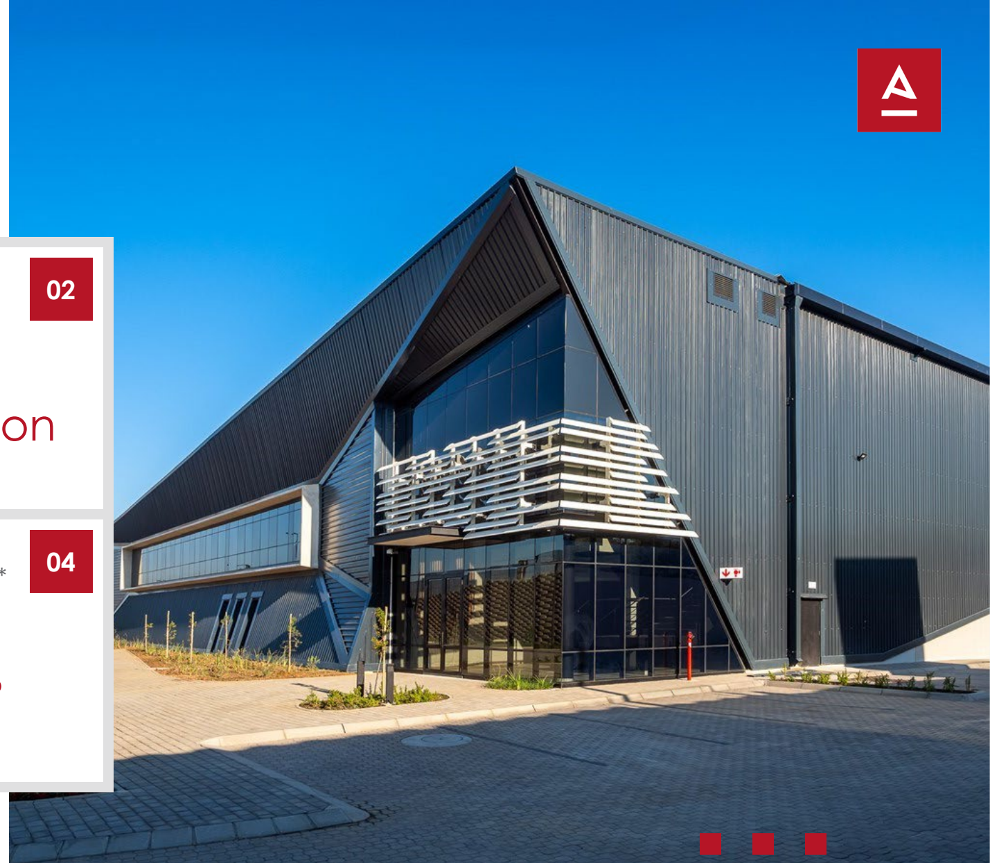
Newly completed midi unit, Waterfall City
