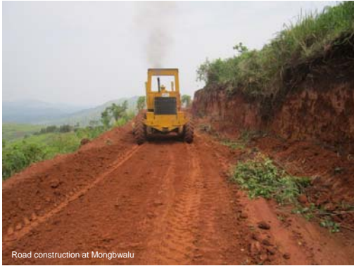
Road construction at Mongbwalu
